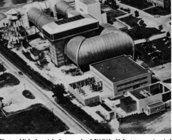
First published aerial photograph of NACA's 16-foot transonic wind tunnel. Tests are made in white building. Drive fans are at far end
